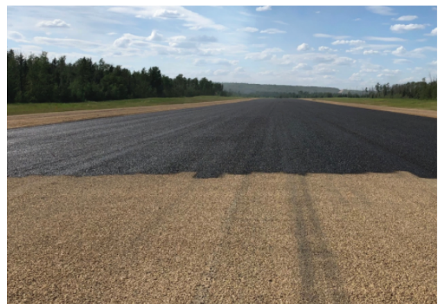
Fog Seal in progress at the Syncrude Airport strip.
