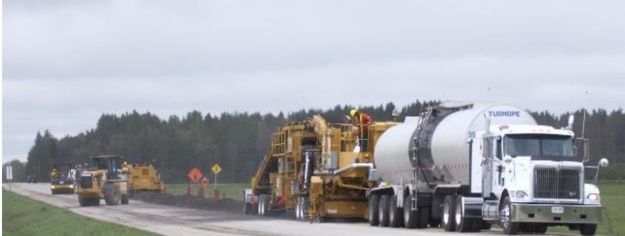
Figure 1. CIR construction recycling existing pavement.
