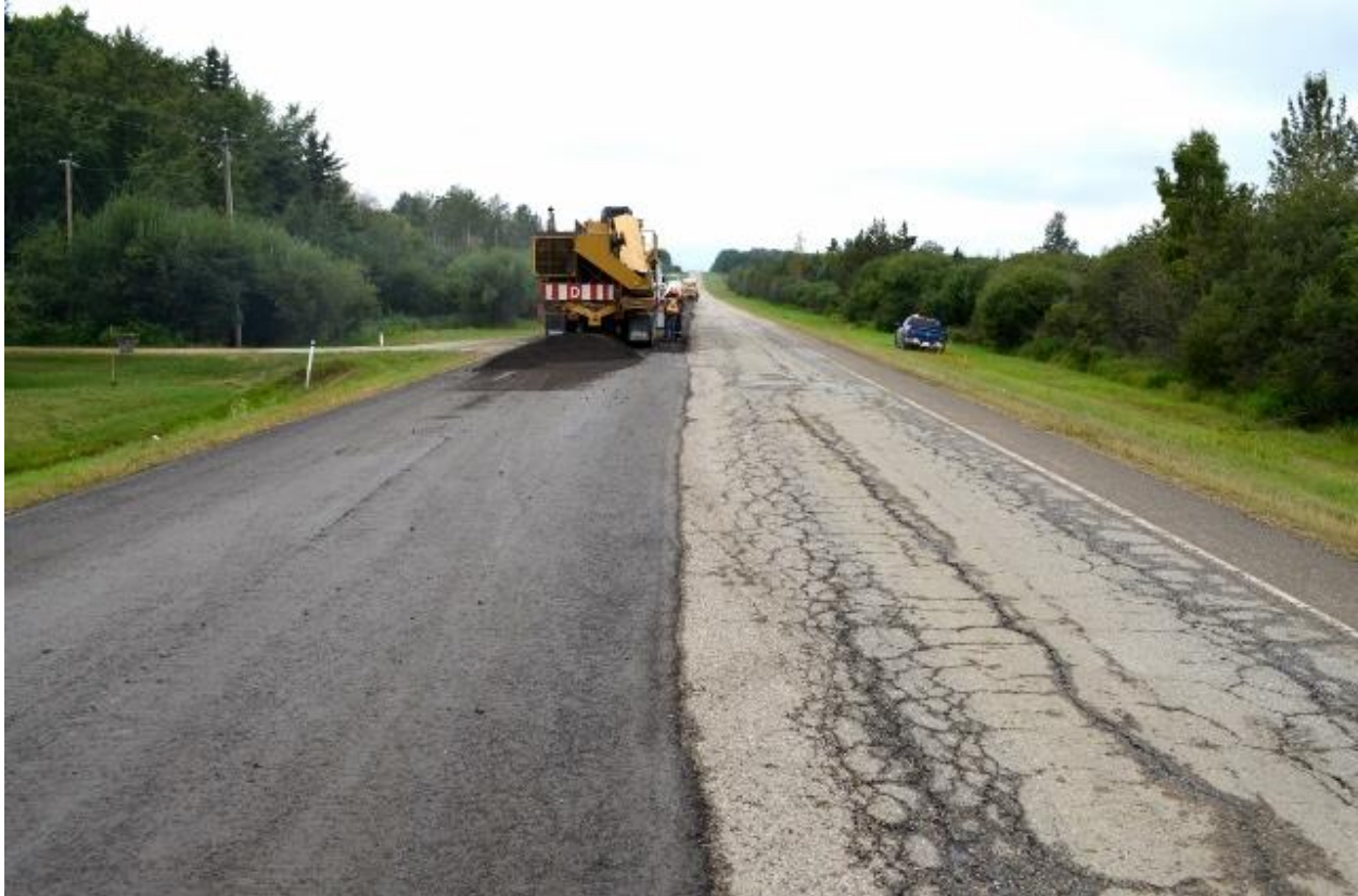
Figure 2. A road which qualified for reconstruction using CIR (Highway 53 near Rimby, Alberta). The right hand lane shows what the road looked like before being recycled.
